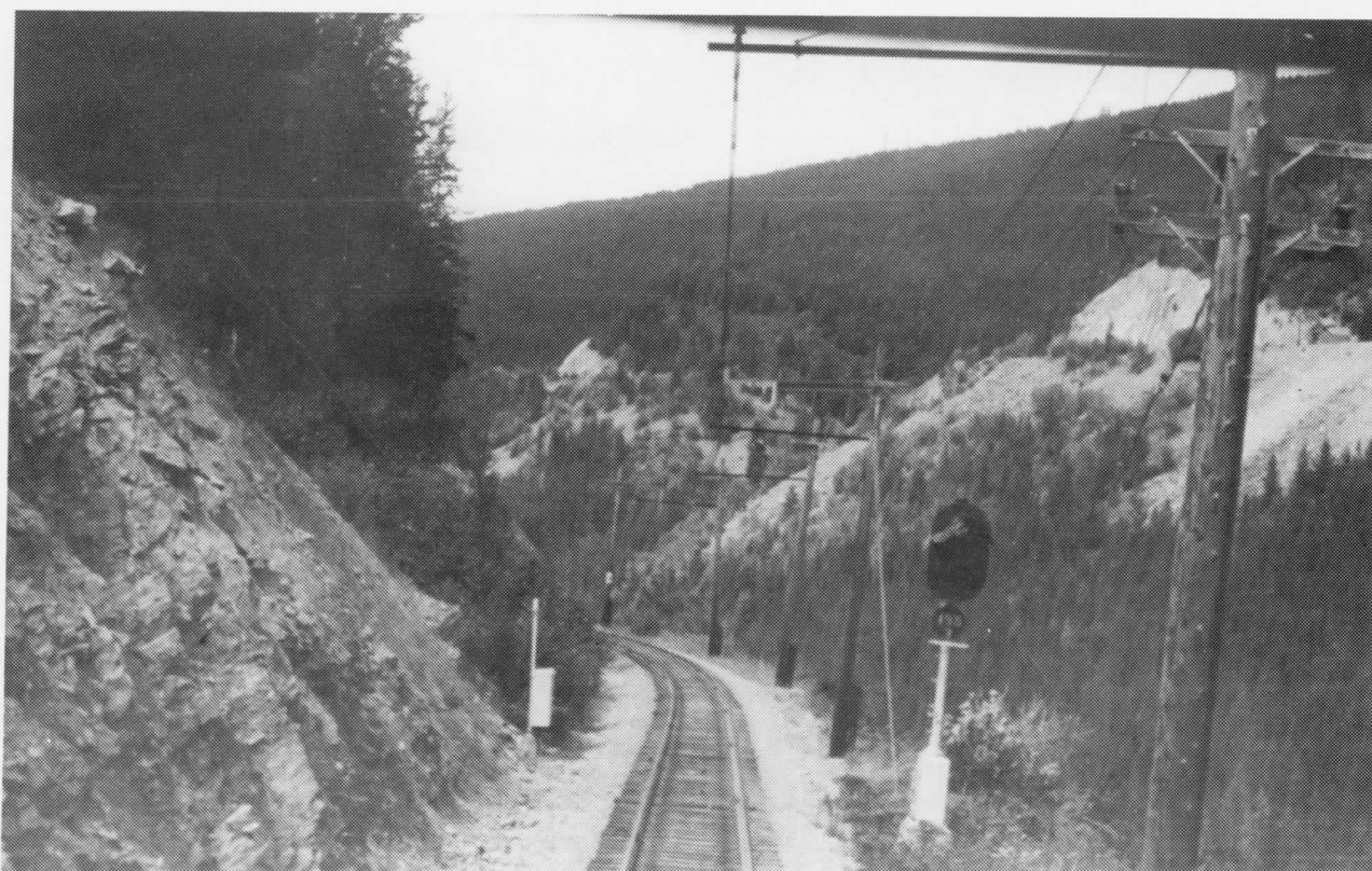
Westbound to Avery. We have just come through the Adiar Loop. The track above is headed to Roland with one of the many steel trestles in this area. Photo - Will Davis collection.
